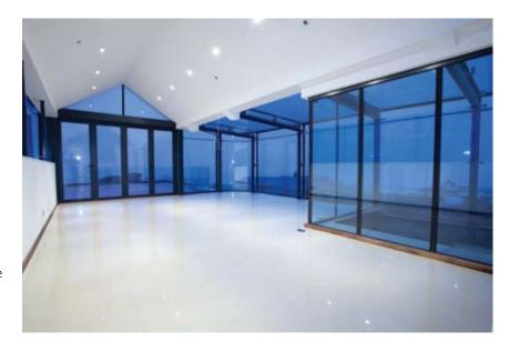
(inner structure) with a spider bolt system connecting the glass. The reason for this was because the Planning Department did not want an outer frame. The glass is double-glazed and provides soundproofing from any other noise in the house and the coastal elements of outdoors.
