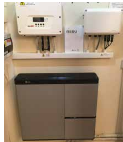
A new installation with LG Battery >
