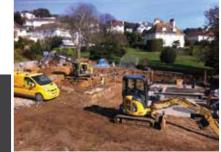
Here you see the formation of the foundation slab for one of the properties ahead of the steel form work and block work.
