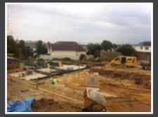
This shows JB Groundworks & Construction completing the dig out for the basement, which they'll then start to lay all the steel in.
